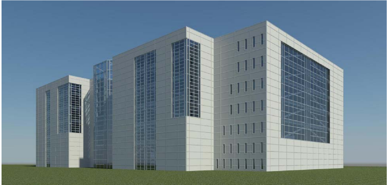
Figure 33: Final Perspective Rendering of CWB with Proposed Composite Steel Framing and Concentrically Braced Frames
