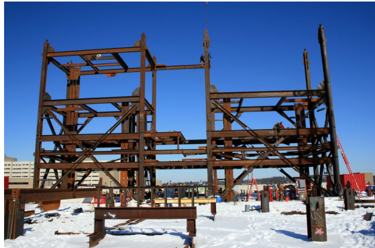
Figure 12: Concentrically Braced Steel Framing (CBF)
